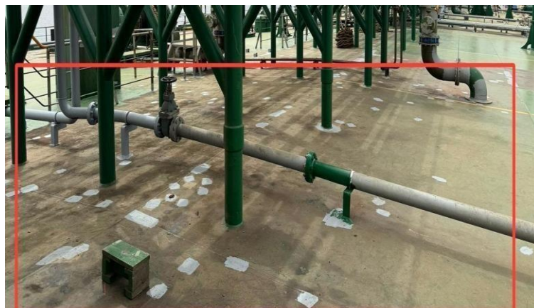
Figure 3. Repaired COW Line Pipe
