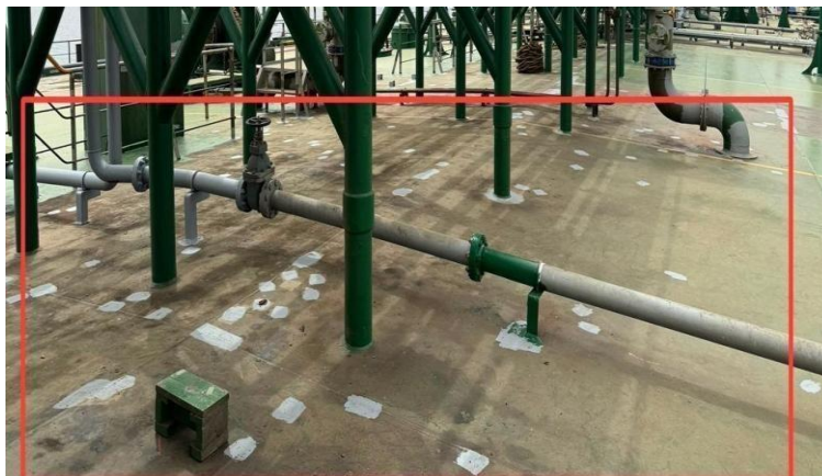
Figure 3. Repaired COW Line Pipe
