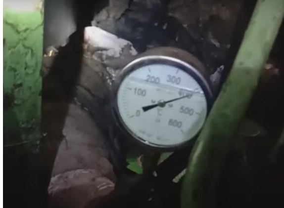
Figure 3. Fuel oil pump
