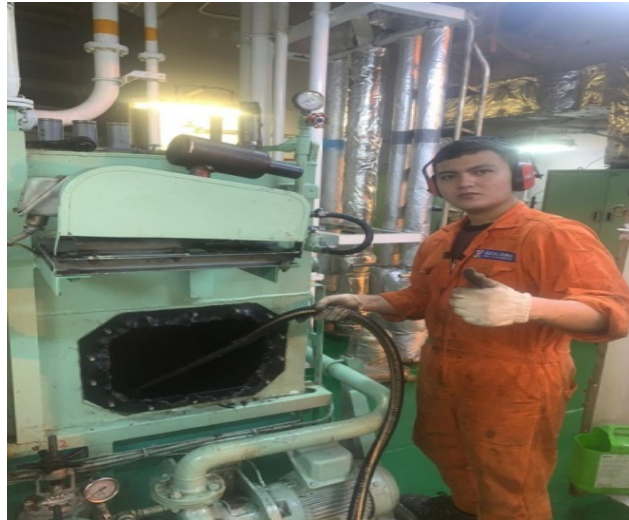
Figure 9. The author cleans the Aeration Tank
